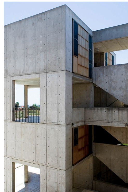
Figure 4: Connections to the 'porticoes of study' via bridges and stairs.
