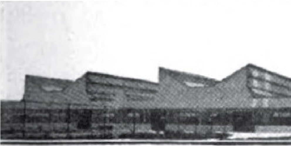
(fig.5) Lincoln plant, showing newer Ford-built addition in rear. (1923)
