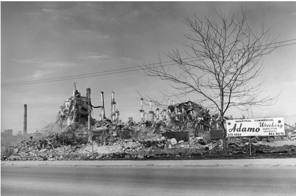
(fig.24) Dodge Main Plant, Detroit. (unknown)
