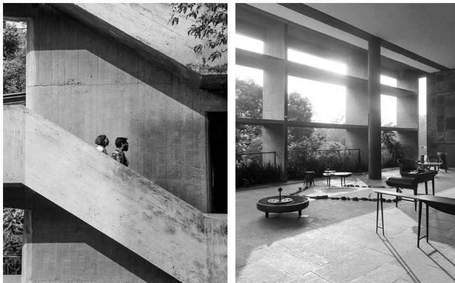
Figure 19 Inside or outside? Stairs are the vehicle to direct people in and out of the building without leaving it.
