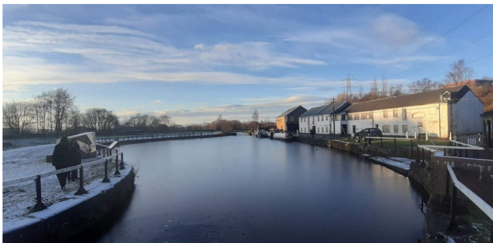
Figure 5 Site of Choice, the workshops at the Hamiltonhill Basin, author's own photo.
