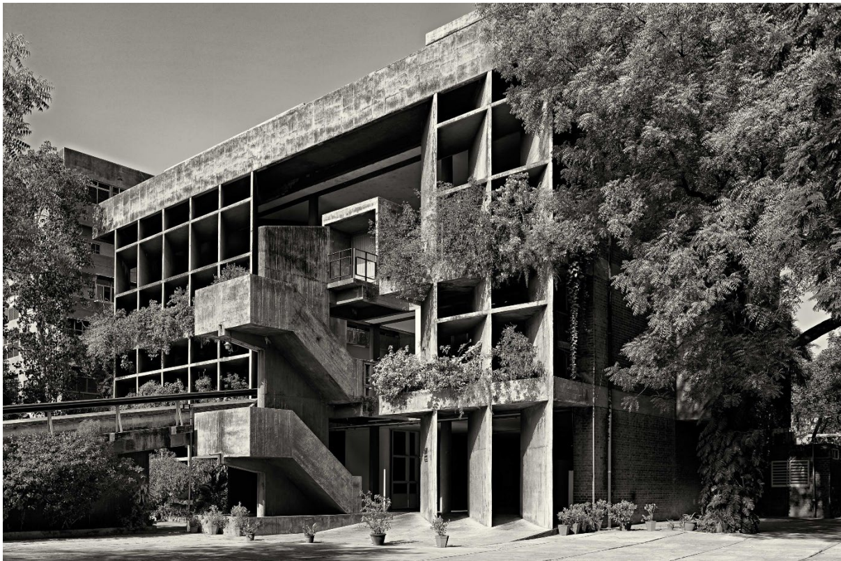
Figure 13 Emden, C. 2017 Le Corbusier Mills Owner Association. Built in 1954, the brise-soleil façade was designed to frame the beautiful views of the surrounding park and the Sabarmati river.
