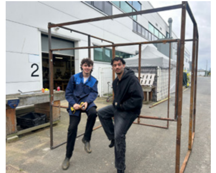
BUILDING THE STRUCTURE
