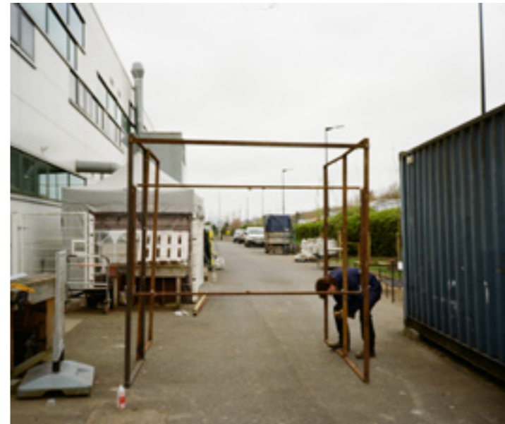
PREPARING THE MODULAR POD
