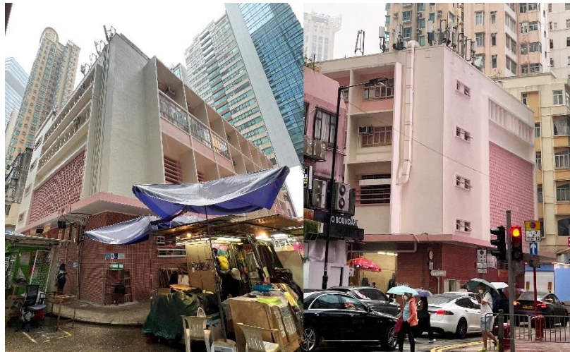
Image 8 & Image 9 Tang Lung Chau Market façade images (Site visited at 18 October 2022)
