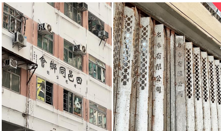
Image 52 Building name signage on Façade image (Site visited at 17 February 2023)
