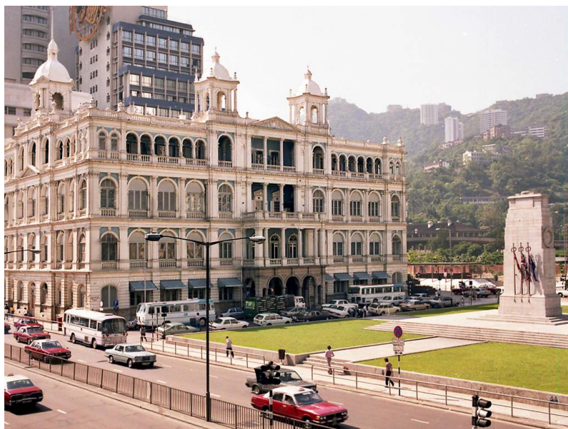
Image 1 Hong Kong Club Building in Central (Demolished at 1981) (Time Out Hong Kong, 2022)
