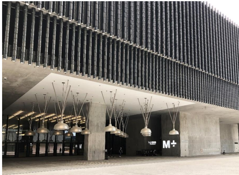
Image 42 Custom terracotta panels of M+ Museum modular cladding system (Site visited at 29 January 2023)
