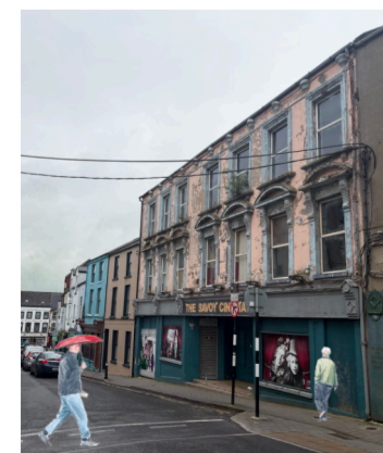
EXISTING BUILDING (West side)
