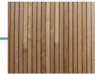
Extension: Western red cedar cladding
