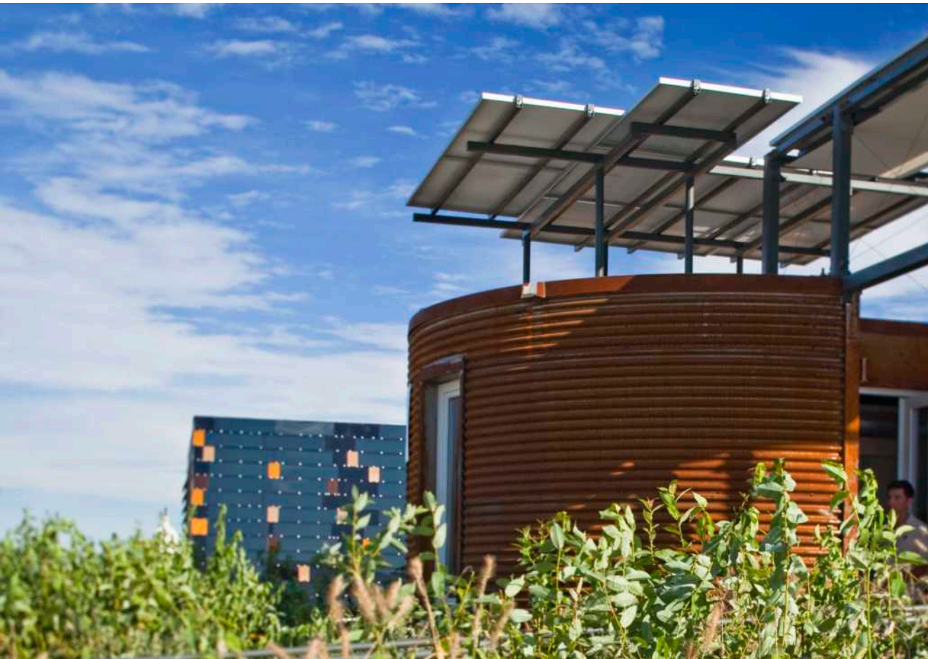
Figure 66 Silo House, Cornell University, One of the Three Living Silos, Ithaca, New York, 2009
