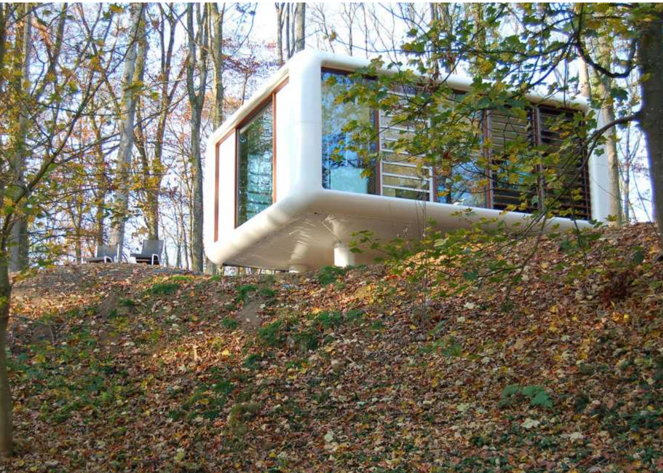
Figure 50 Loftcube, Studio Aisslinger, Berlin, Adaptability, Chatau Poste, Belgium, 2014
