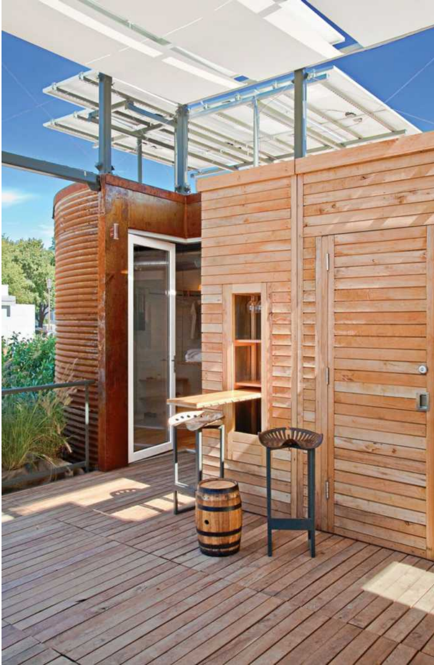
Figure 73 Silo House, Cornell University, Exterior Material and Process Benefits, New York, 2009
