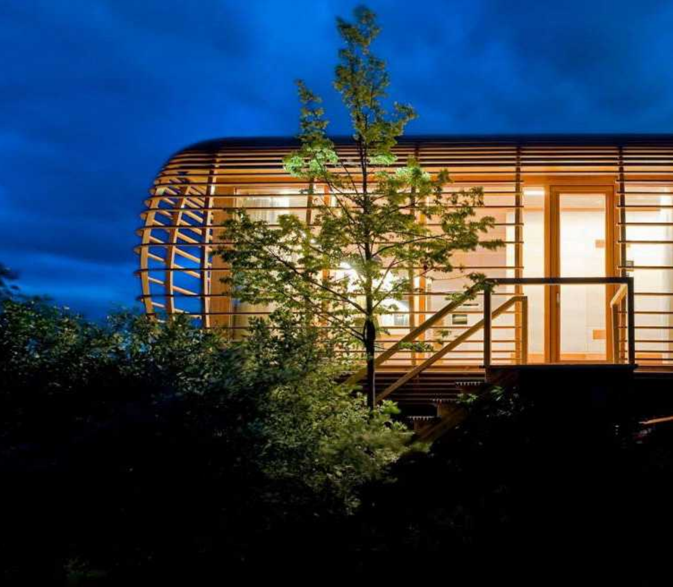
Figure 82 Fincube, Studio Aisslinger, Off-Grid Electricity Use, Ritten, Italy, 2010
