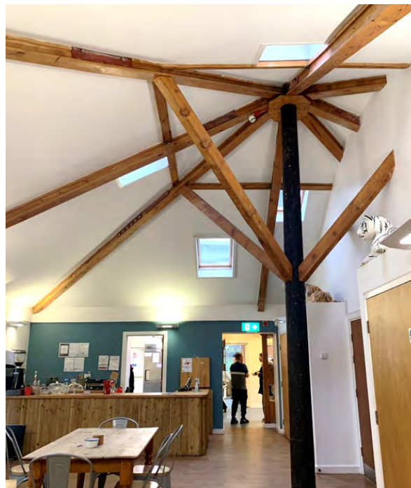
39. VAULTED CEILING FROM ORIGINAL BUILD
