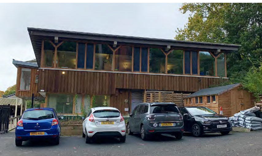
30. EAST FACADE & STAFF PARKING
