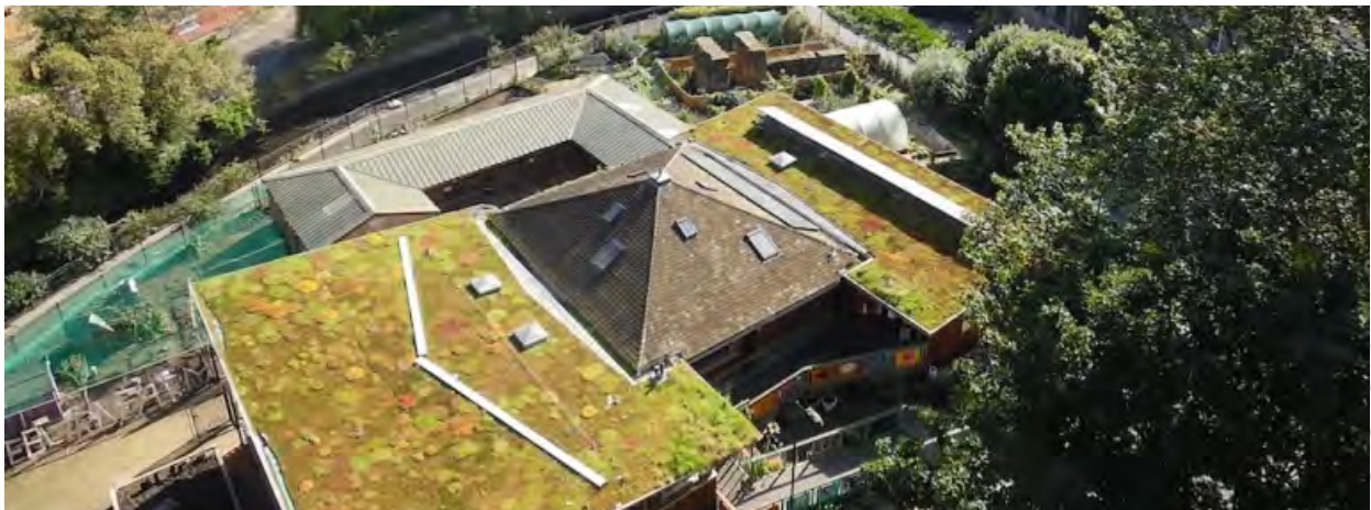
32. VIEW OF SEDUM ROOF & SOLAR PANELS
