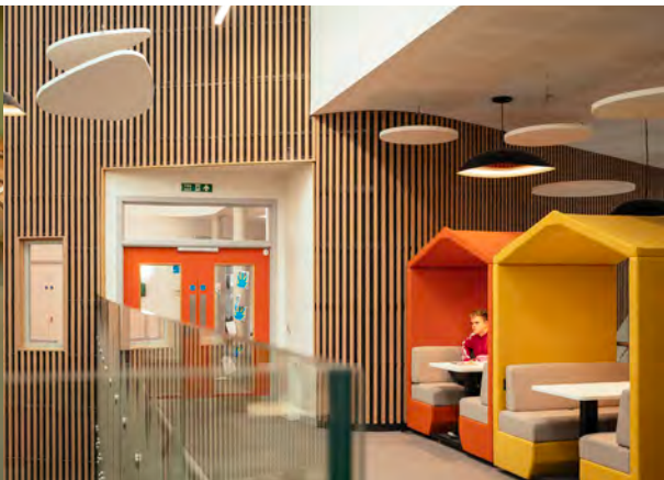
Image 6 Wooden cladding to control acoustics (eliminate unwanted vibrations) – semi-private self study pods still providing views. (Astbury, 2023)
