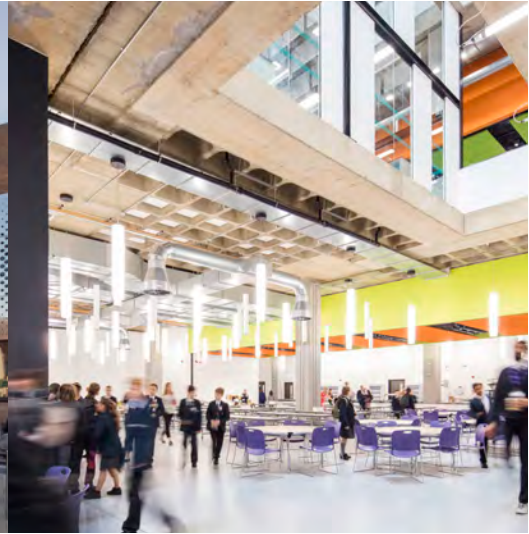
Image 29 Exposed existing waffle slab integrated within the new design (Tapia, 2019)
