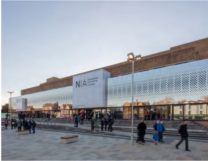
Image 28 Image displaying the clear difference between the old and the new (existing building and new facade) (Tapia, 2019)
