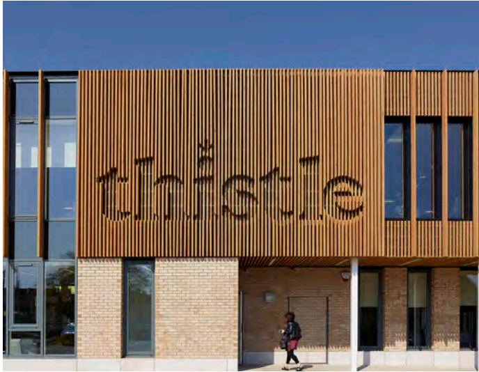
Image 24 Image displaying clear signage integrated into external timber cladding – clearly defining entrance of the building (Cardenas, 2016)
