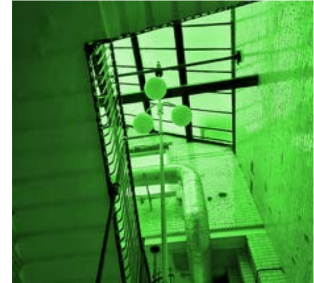
Staircase to get to the Flat Roof
