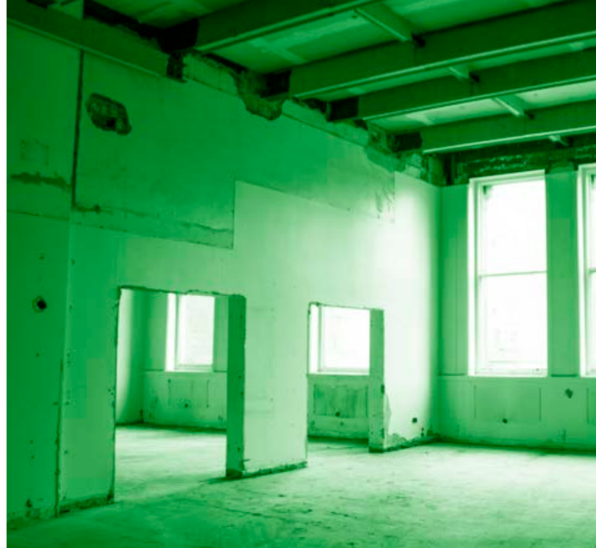
This images shows the solid Masonry walls
