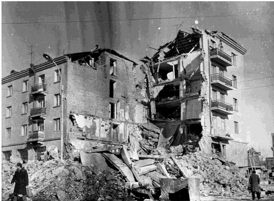
FIGURE 5. AFTERSHOCKS OF THE DESTRUCTIVE EARTHQUAKE DESTROY MORE HOUSES.
