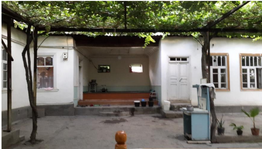
FIGURE 1. TRADITIONAL UZBEK HOUSE WITH A COURTYARD. INNER WALLS MADE OF MUDBRICKS WITH A LAYER OF CLAY.
