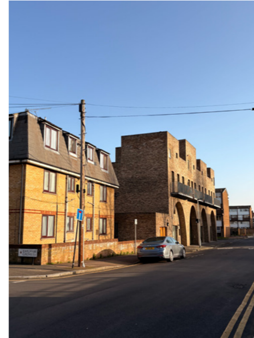
Figure 27: McGrath Road street view with surrounding context
