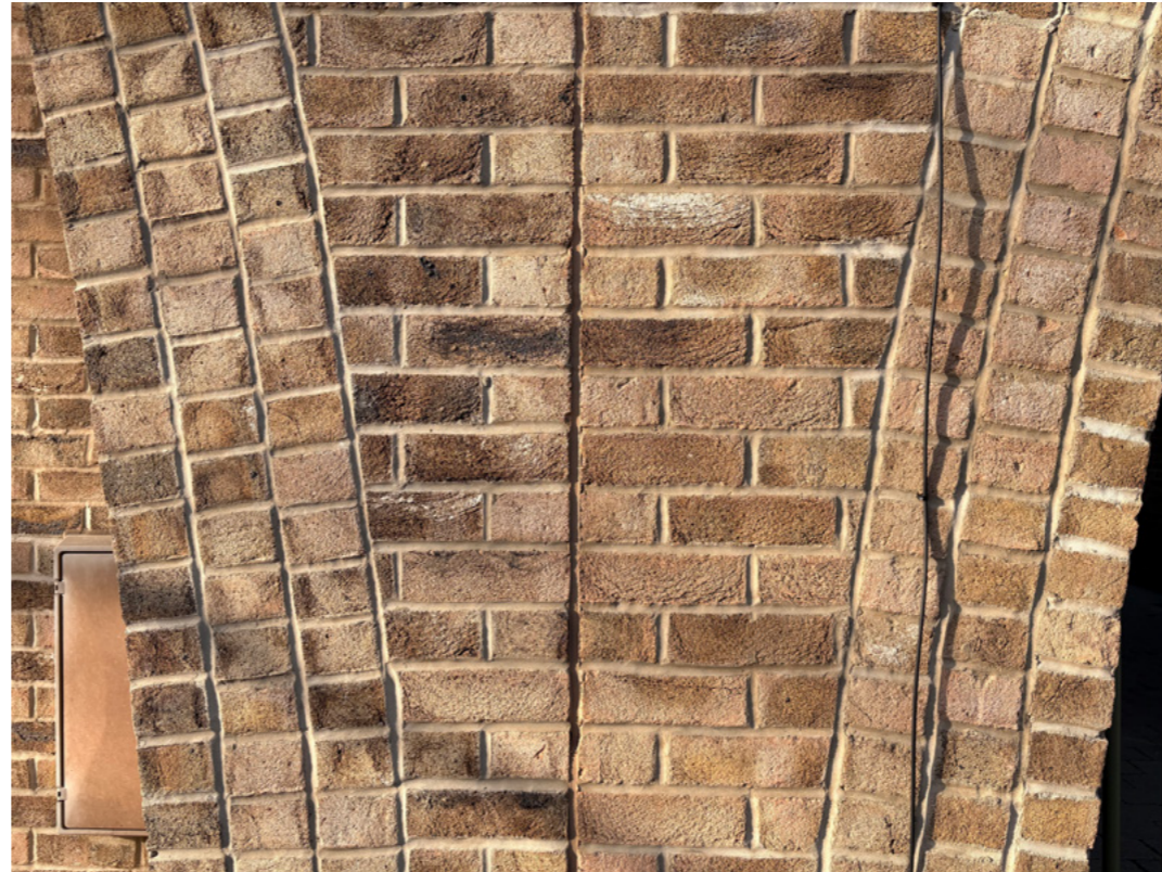
Figure 44: Brick joint and material detail
