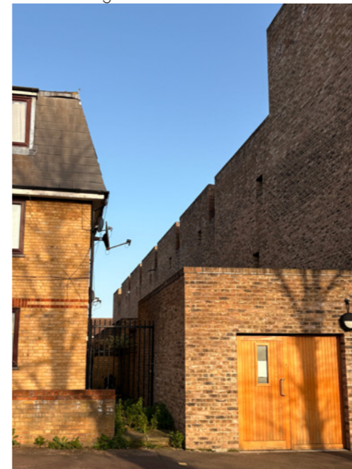
Figure 30: Tower house facade detail
