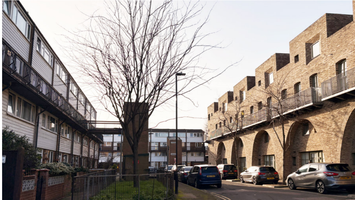
Figure 26: McGrath Road street view with surrounding context
