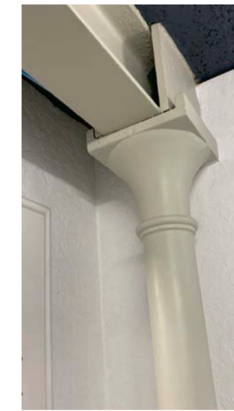
Steel Column Structure
