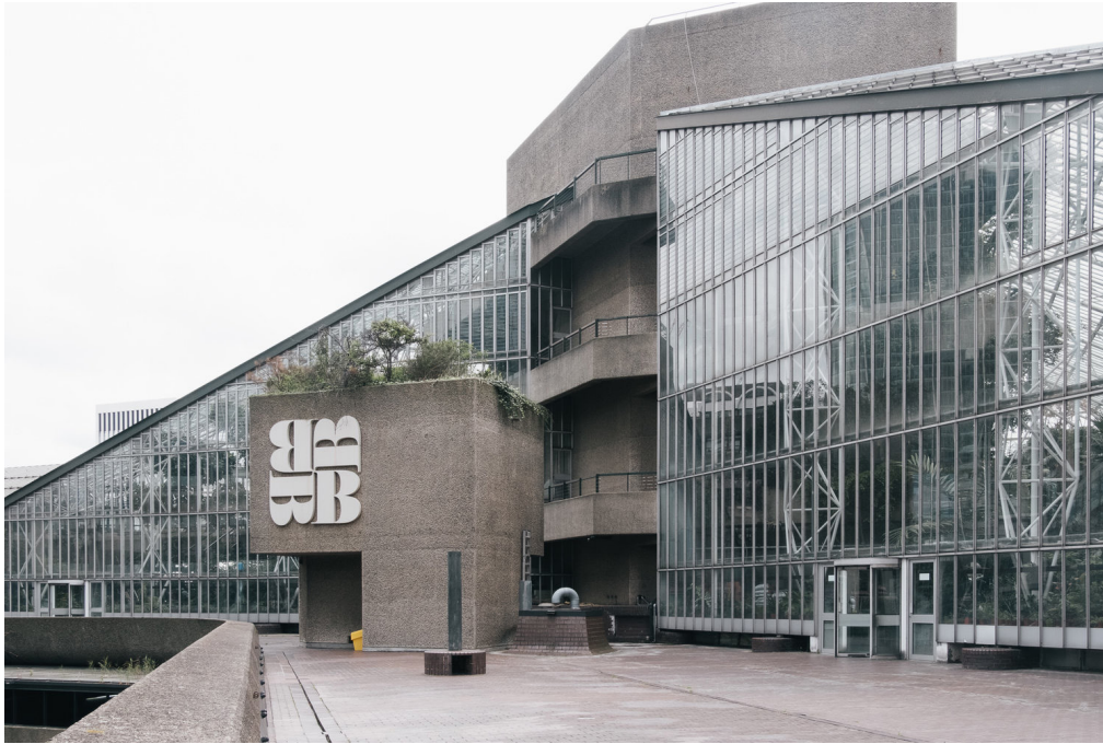
Fig 15. The external perimeter of the Conservatory forms the connection between the brutalist concrete architecture and the lightweight glass facades.
