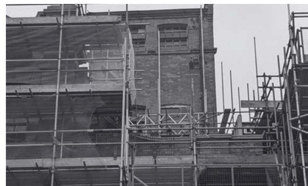
FIGURE 30: BREWERS QUAY SITE VISIT #3 - EXTERNAL HERITAGE DETAILING
