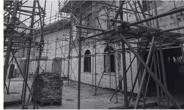
FIGURE 28: BREWERS QUAY SITE VISIT #1 - RESIDENTIAL MEWS
