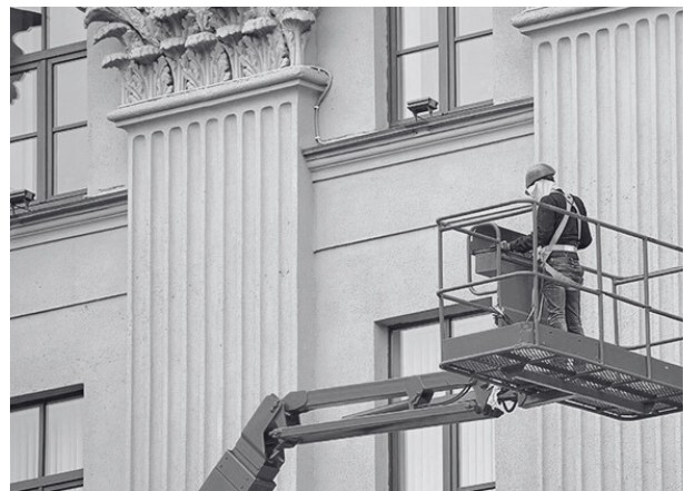
FIGURE 14: PRESERVING THE PAST, ADAPTING FOR THE PRESENT: THE USABILITY CHALLENGE IN HERITAGE CONSERVATION
