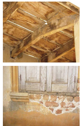
Figure 12 Evidence of decay: broken joists and peeling wall plaster
