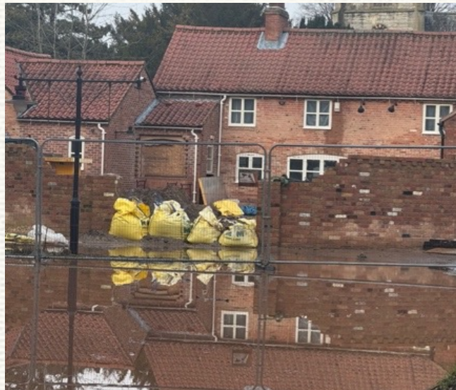
Figure 21 | A photo taken of 'The Beck at Cauntton' showcasing the newly built wall as a flood preventative.
