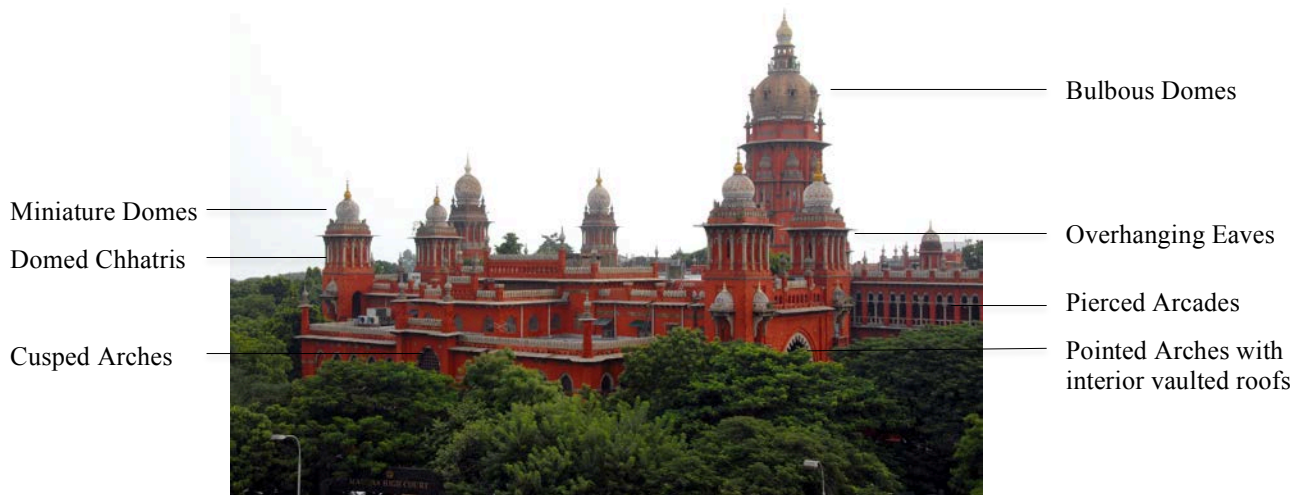
Figure 10: A famous example of Indo-Saracenic Architecture - 'Madras High Court', Madras (modern day Chennai)
