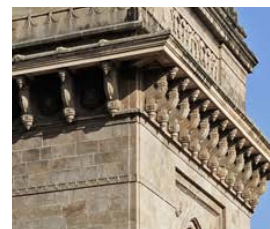
Chhajjas (Overhanging Eaves)
