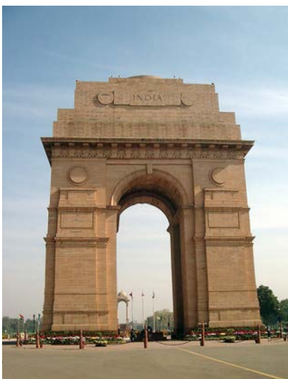
Figure 17: 'India Gate'- Designed by Edwin Lutyens
