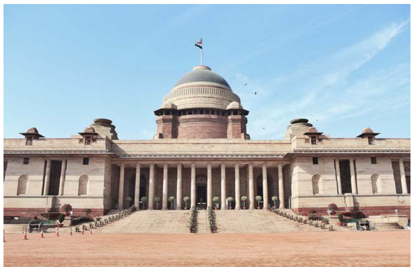
Figure 18: Rashtrapati Bhavan – The Viceroy's (President's) House- Designed by Edwin Lutyens
