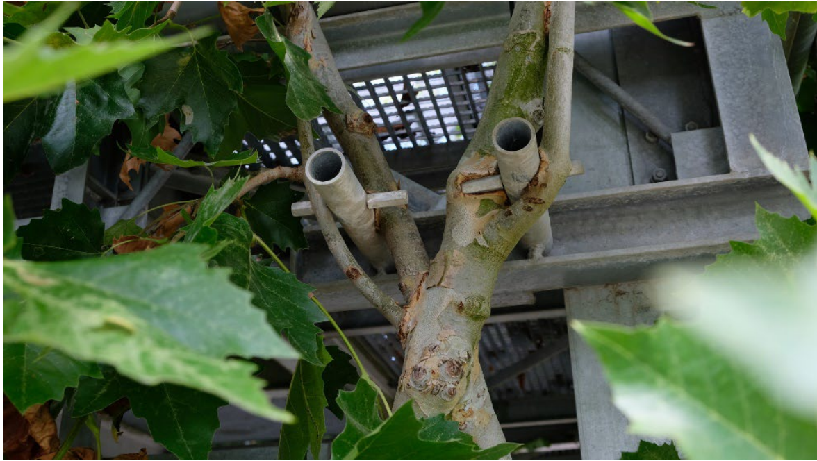
Figure 16 Close up of steel frame and trees intersecting
