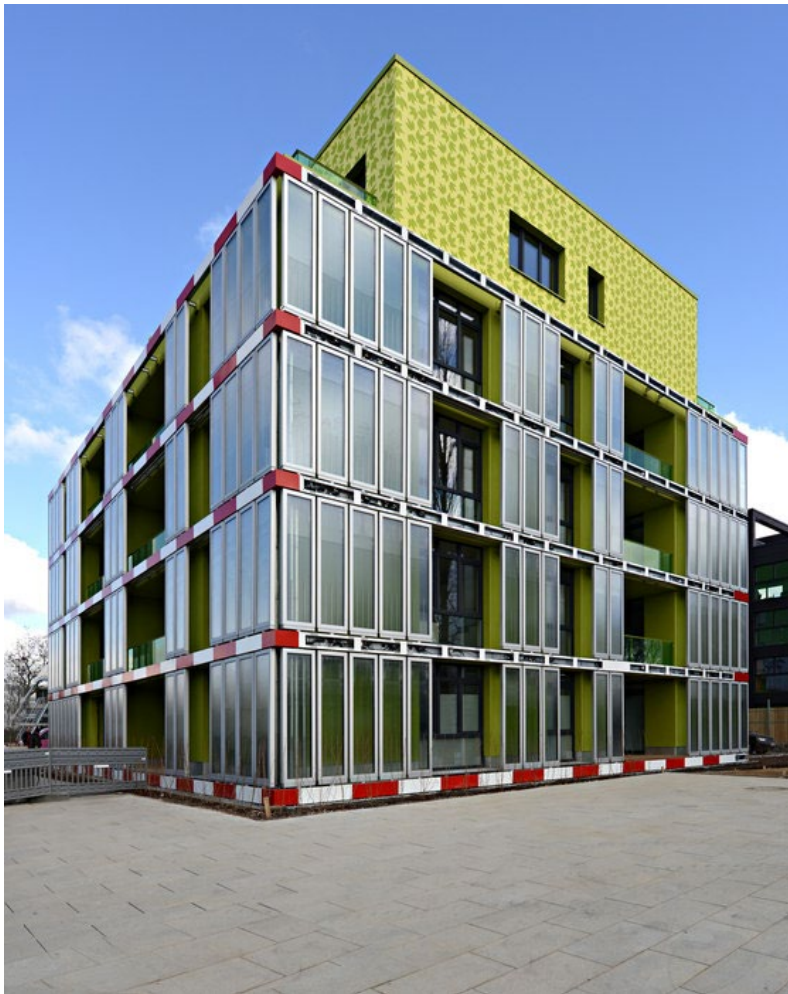
Figure 6 Bio-reactive facade on BIQ House
