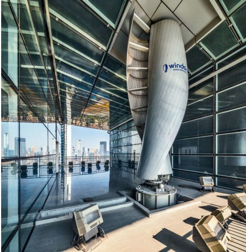
Figure 13 Vertical wind turbine within one of Pearl River Tower' s envelopes
