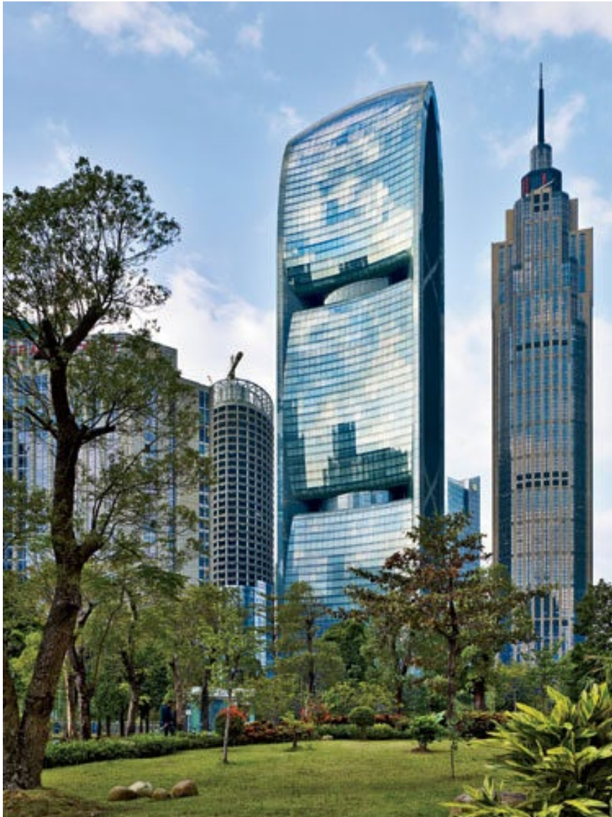
Figure 14 Exterior of Pearl River Tower
