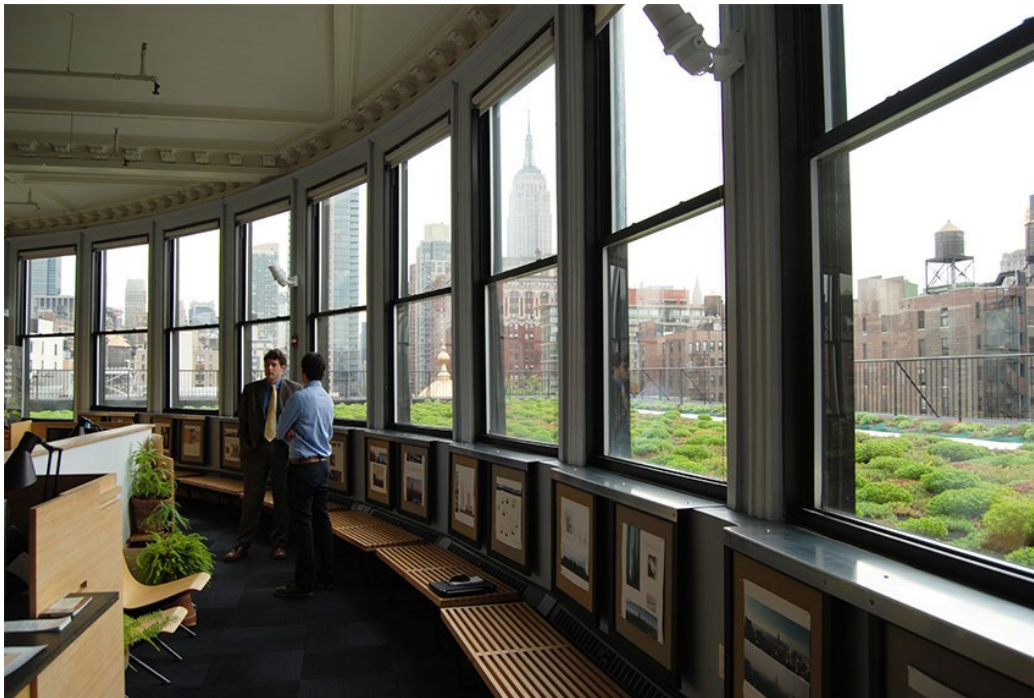
Figure 8 Northeast wall looking over green roof
