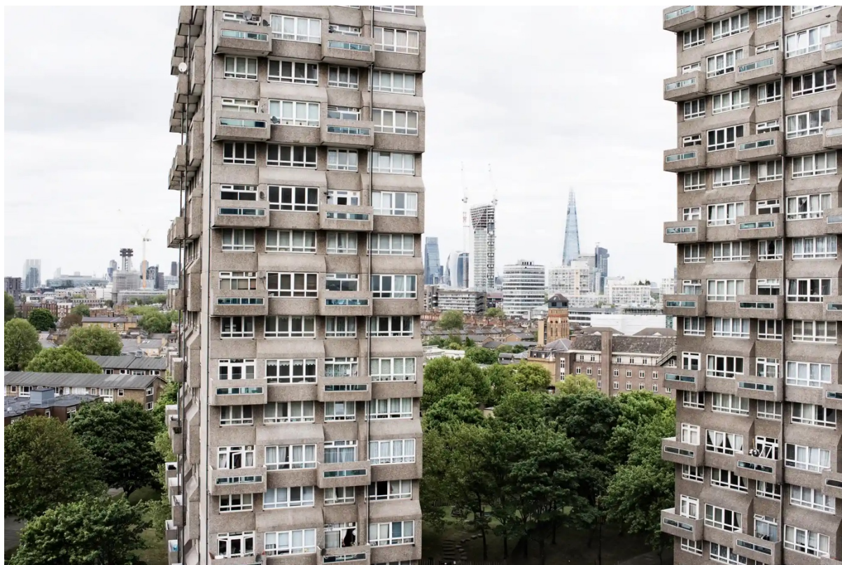
Fig 1: 1950's Mass Housing Hidden in Plain Sight, Surrounded by the Denial of the Public.
