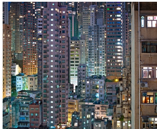
Fig 28. Hong Kong's Dense Tower Blocks
