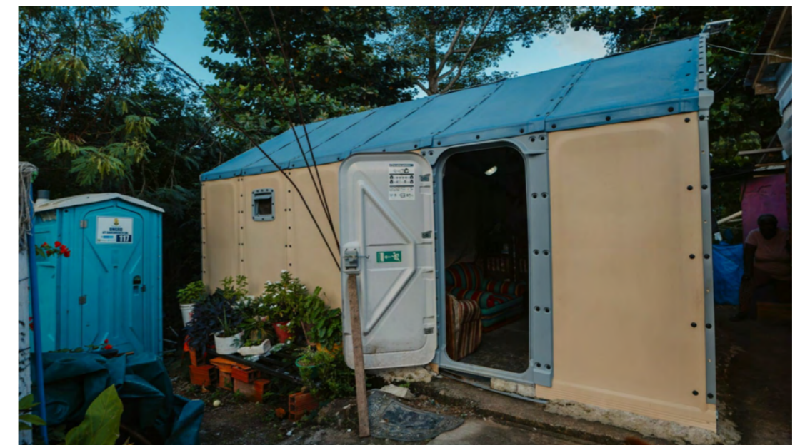
Figure 5 Hagman. E. (2016). Interior of a Shelter in Iraq. [image] Available at: https://www.theguardian.com/artanddesign/2017/jan/27/why-ikea-flatpack-refugee-shelter-won-design-of-the-year (Accessed 15 November 2023)
