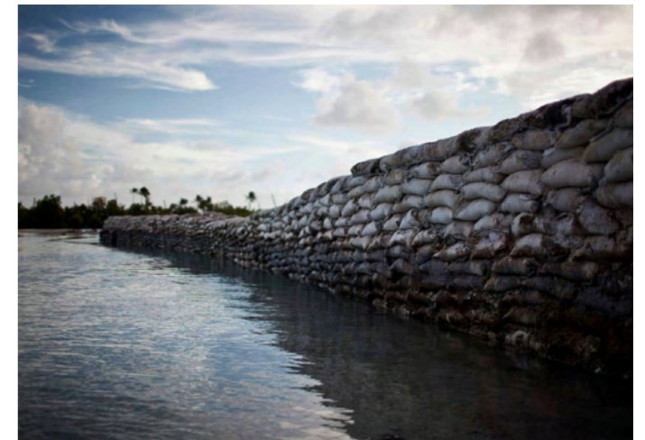
Figure 36. Jazbec, C (n.d) A sea wall in Maneaba, Kiribati to protect buildings from flooding. [Image] Available at: https://www.globalonenessproject.org/library/photo-essays/kiribati-gone#photo-12=&sm=pe21520.8573&info=true (Accessed 15 January 2024)
