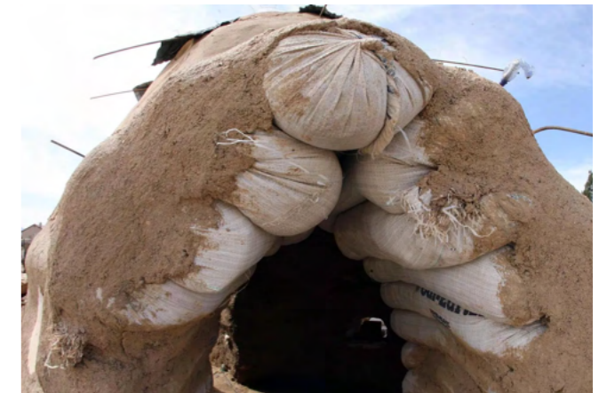
Figure 16 BBC Future. (2019) The process of making the Superadobe. [Image] Available at: https://www.bbc.co.uk/future/article/20190228-what-is-superadobe (Accessed 29 December 2023)
