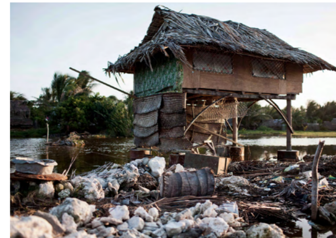
Figure 35. Jazbec, C. (n.d) A house lifted and placed on stilts in Tarawa, Kiribati to prevent flooding. [Image] Available at: https://www.globalonenessproject.org/library/photo-essays/kiribati-gone#photo-12=&sm=pe21520.8582&info=true (Accessed January 15 2024)
