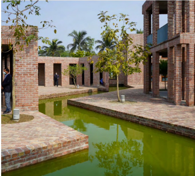
Figure 7 Hossain.S. (2022). The rain harvesting canal that separates the hospital in section and acts a protective barrier against flooding. [image] Available at: https://www.aljazeera.com/gallery/2022/11/31/pictures-world-best-new-building-bangladesh-friendship-hospital-riba-award (Accessed 13 November 2023)
