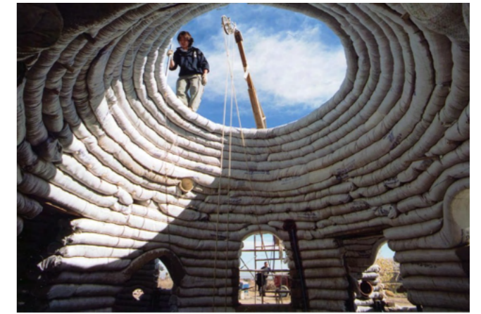
Figure 15 Cal-Earth (n.d) Construction of Superadobe. [Image] Available at: https://www.calearth.org/intro-superadobe
