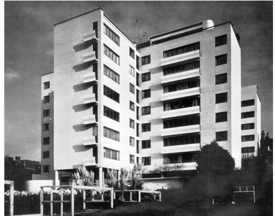
Fig 32. Apartment Block 'Highpoint I' by Tecton in London, England (Dell & Wainwright, 1935)
