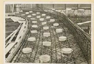
RAMPS IN CONSTRUCTION
