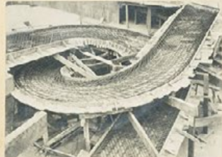
ROOF IN CONSTRUCTION
