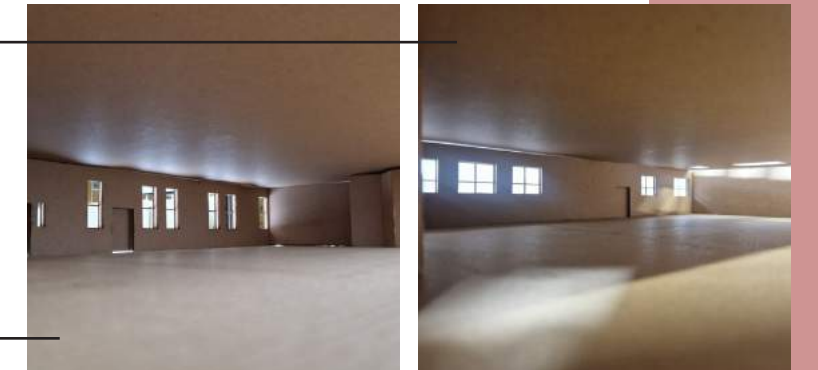
Ground floor - Southwest
