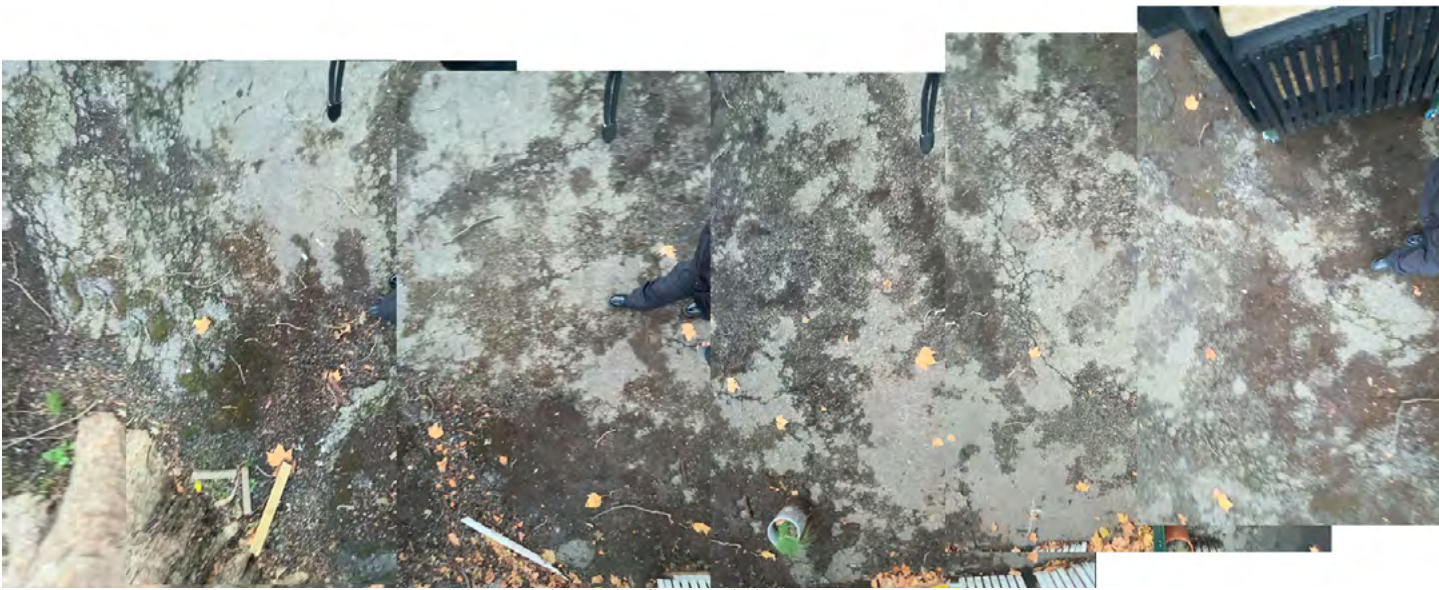
Cracks on the floor made by tree roots.
