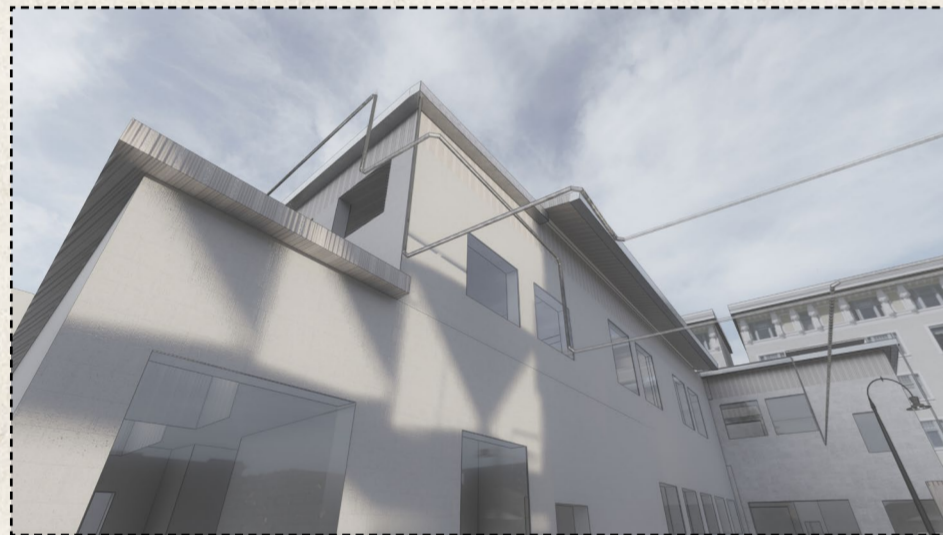
"This is the pipe that collects rainwater!"
