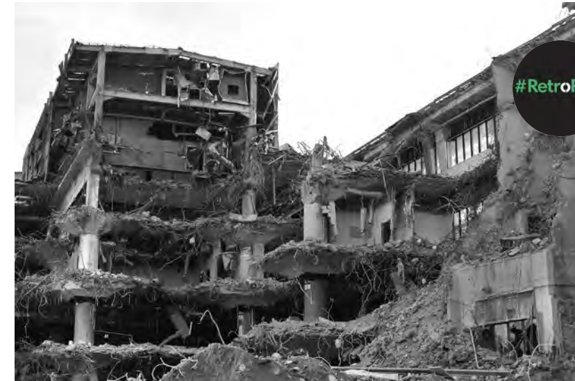
Demolition of an old building with floors
