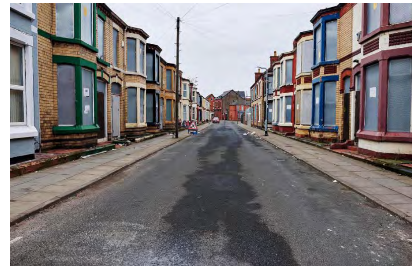
Boarded up houses in Granby area of Liverpool
