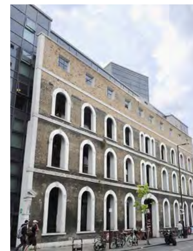
Façadism on Caledonian Road, Islington
