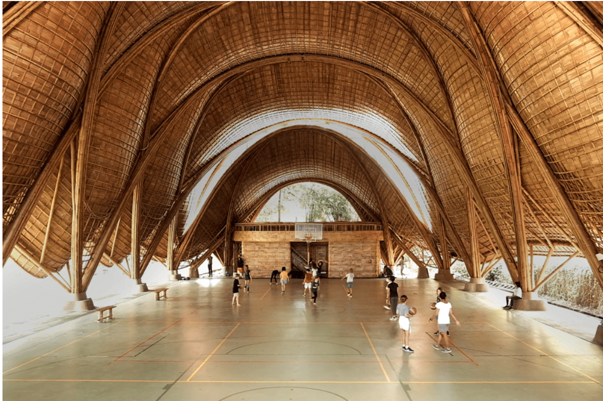
Fig 2.2 - The Arc, the gym hall at the world renowned Green School in Bali, Indonesia. The difficult design task of creating an unprecedented inner volume with an impossibly thin structure, without any disturbing trusses found its answer in nature; the human ribcage.
