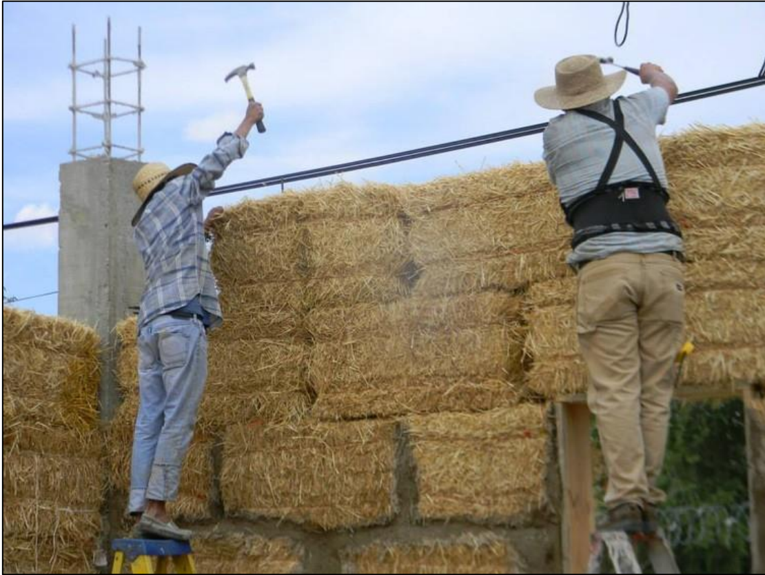
Figure 2: Construction of the chapel by locals (Chopeke, 2018)
