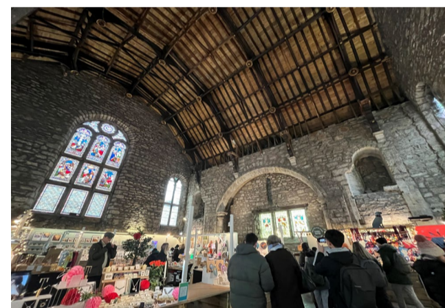
Existing hammer-beam ceiling
