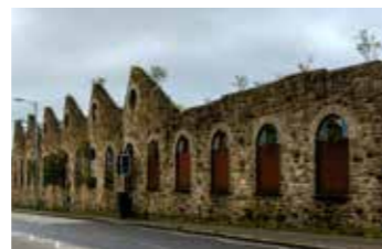
Northlights building in disrepair.
