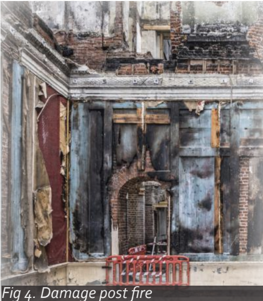
Fig 4. Damage post fire
