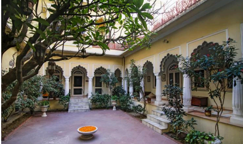
Figure 13 ( Top ) - Common rajasthani haveli chowk, this one is in a heritage hotel.
