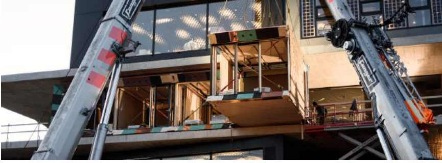
Figure 12 (top left) Prefab unit being built off-site.
