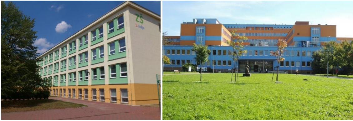
Fig. 2: (left) Renovation of Primary School with colourful façade
