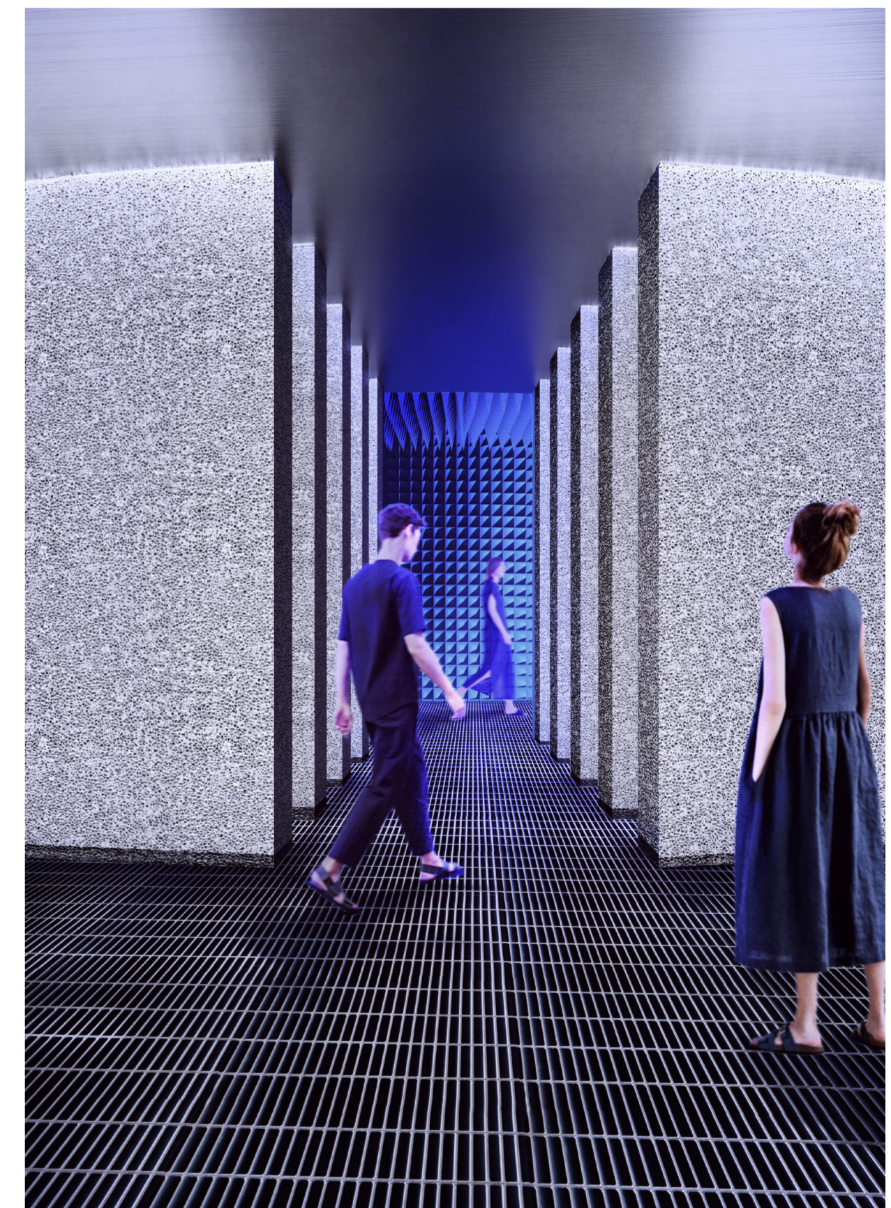
Above: Approach to anechoic corridor with large panels of aluminium foam layered to form acoustic barrier. Opposite: Entrance to acoustic corridor where walls and ceiling are lined with carbon loaded polyurethane.
