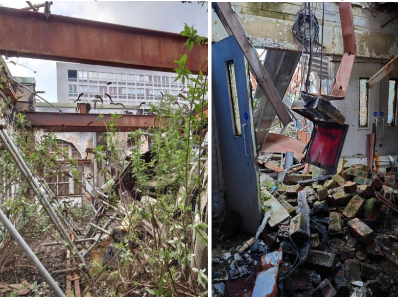
Views showing the collapsed interior and fire damage.
