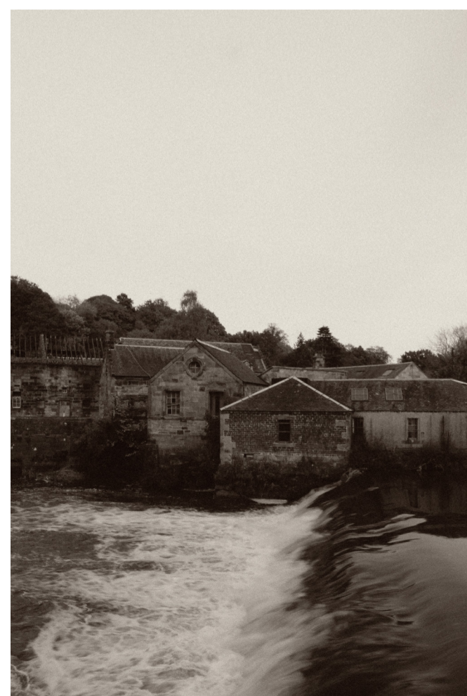
Weir's cascade, March
