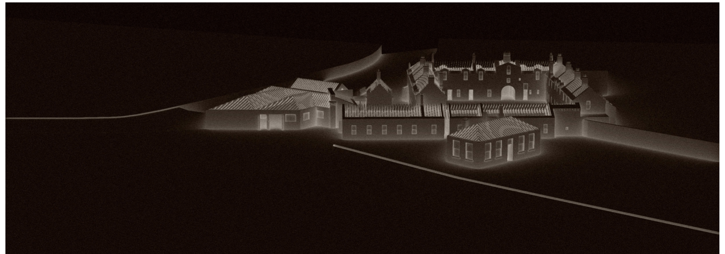
Exploring Roof Structures
