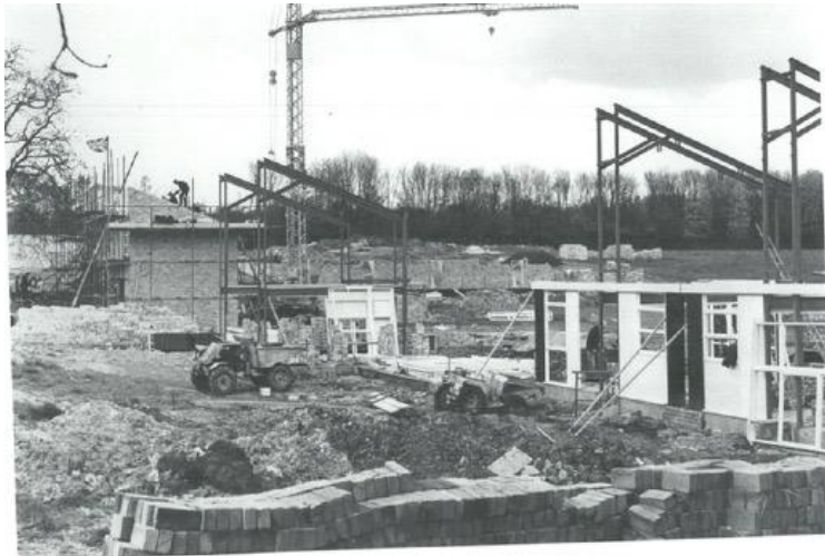
Figure 2: Simms, B. Construction of First Houses on Over Minnis (2006)
