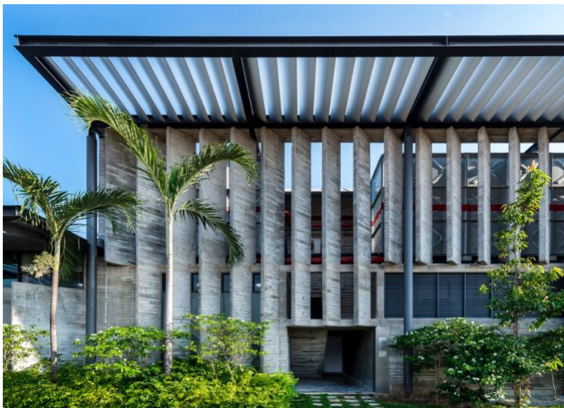
Figure 13: Ho, L. Factory in the Forest Natural Ventilation (2017)
