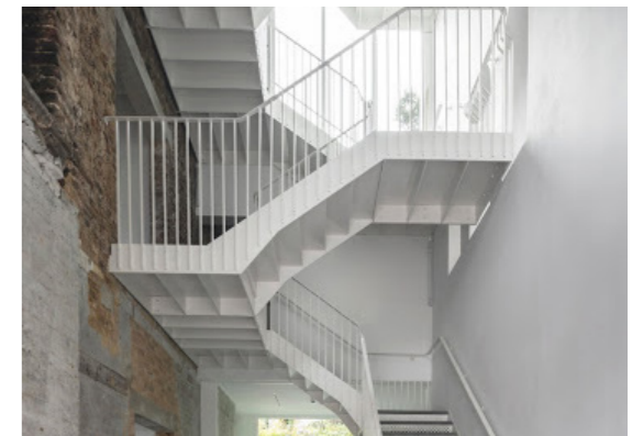
Photograph of staircase at SLG Fire Station
