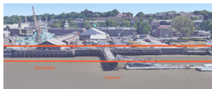
Floodwall along The Medway in Chatham
