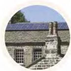
Removable Solar Panels - 150mm stand off above stone slate roof.
