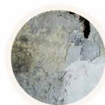
8. Traditional Lime Render - peeling and cracking due to age and sun exposure through windows & openings.
