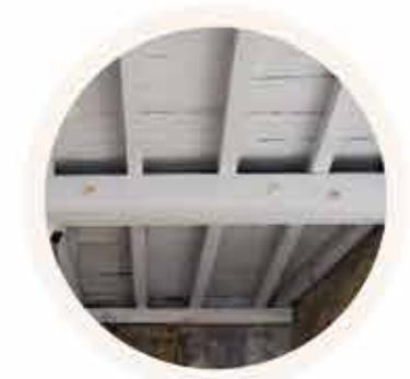
6. Change in ceiling - exposed beams, joists and timber floorboards above.
