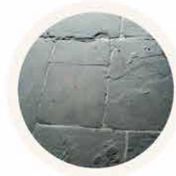
4. Stone Flag Floor - newly insulated & re-pointed on a lime mortar bed.
