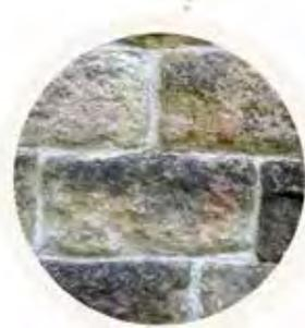
Stone Walls & lime mortar in a semi-regular running bond pattern.
