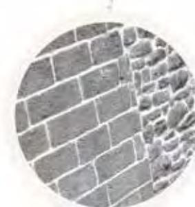
Different stone has been used to repair entrance into weaving shed.
