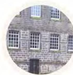
Lime Mortar - Colour variation due to repair work throughout exterior.
