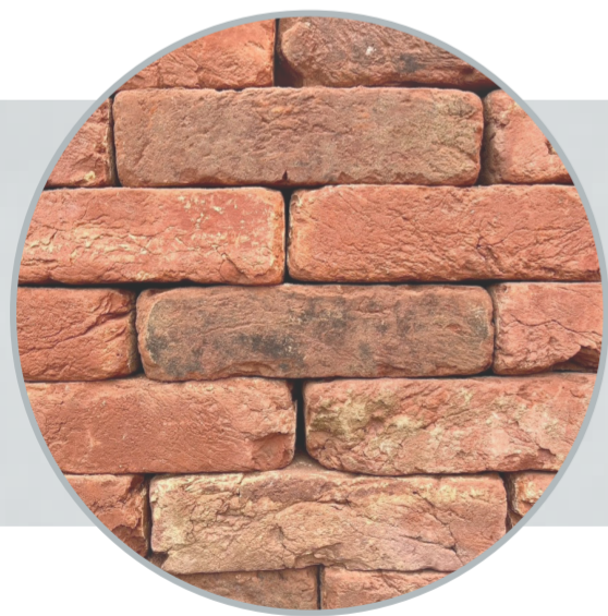
Existing red brick exposed
