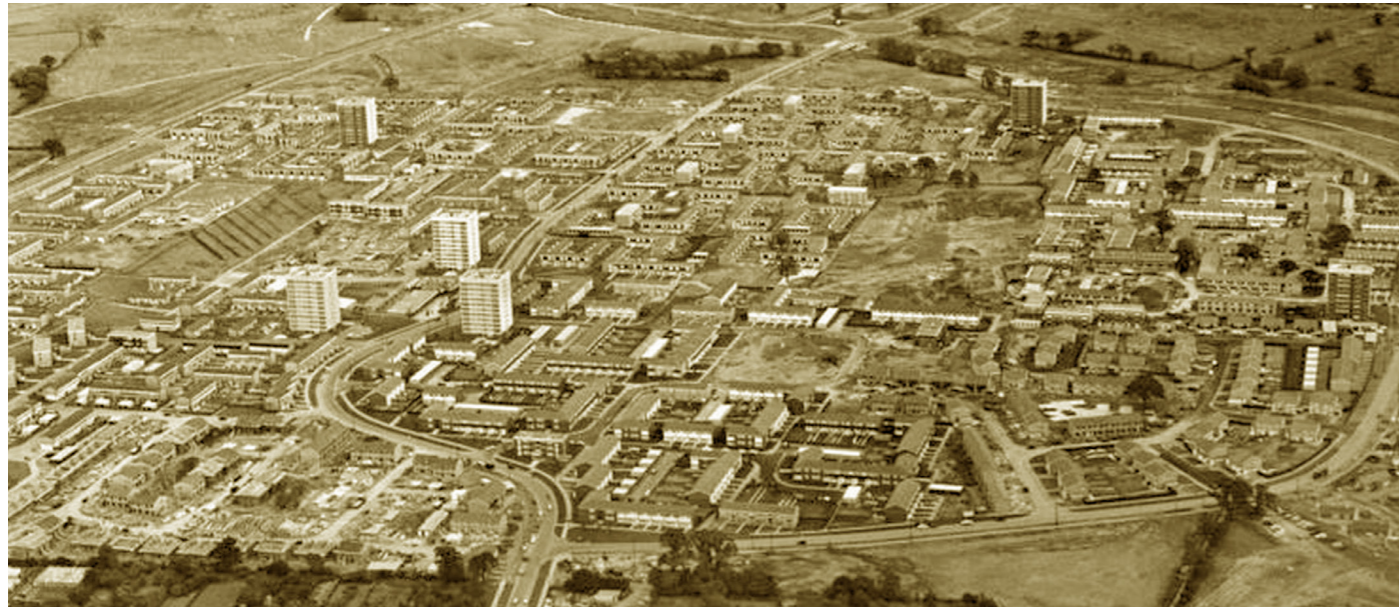
Figure 5: Chelmsley Wood Estate showing an aerial view of the whole estate when it was first opened in 1960 (BirminghamLive, 2014:online)
