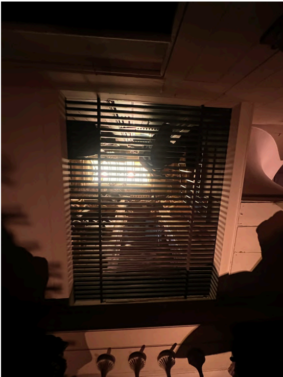
Fig 20. Photo showing perforated floor placed create dim lighting on floor below. Photo by Hammoud, F
