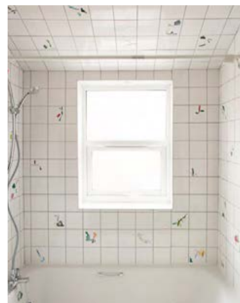
Figure 50: Tiles installed in bathrooms.
