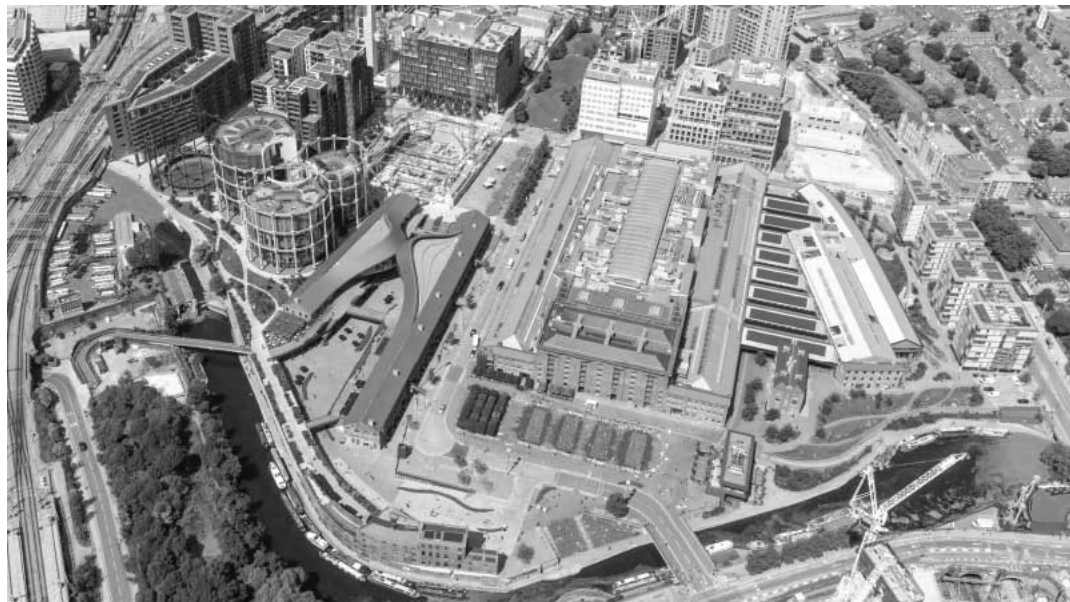
Fig 18. The Montifraulo (2012) The newly completed King's Cross Square
