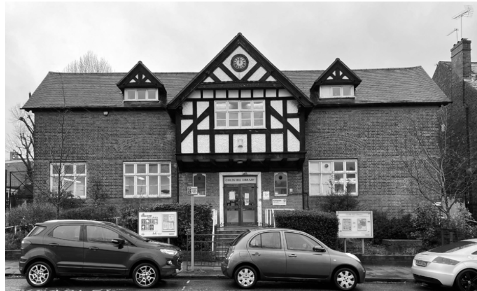
Street view of the site.
