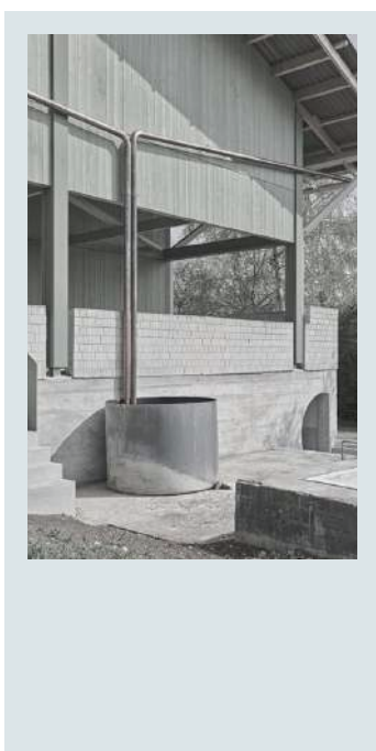
Rainwater being collected through the roof gutter into the basin placed down.
