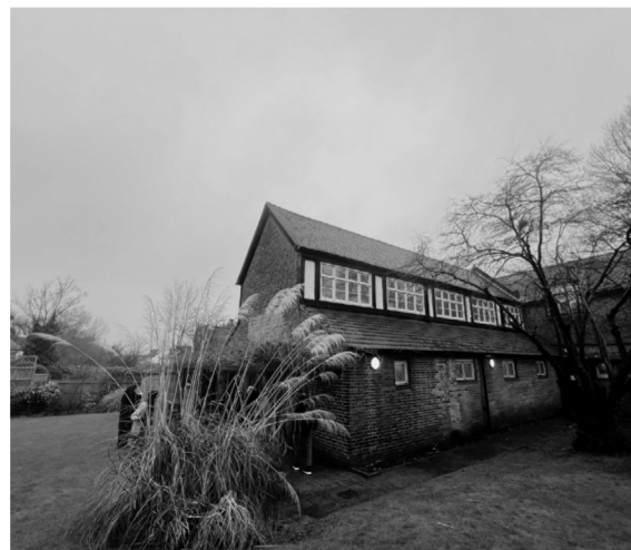
On the back of the building a garden surrounds the library and create an open space.
